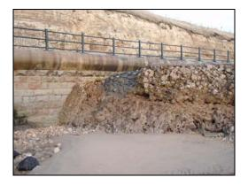
South of Parson's Rocks the defence is a masonry seawall with a concrete block crest (pictured, right). The crest level of the structure varies. The masonry is generally in good condition although several blocks are cracked and in need of repair. Repointing should be carried out to replace missing mortar which is particularly evident in the lower, intertidal section of the wall.
