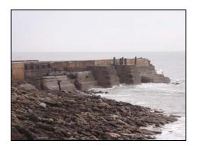
Significant erosion had taken place to the seaward face of the structure, with displacement of large concrete blocks and steel piles exposed and badly rusted. Although the toe was not visible due to the water level, the visible section of the wall was displaced in a manner which suggested undercutting of the toe of the pier was occurring.
