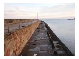
A concrete crest wall runs along the centre of the structure and appeared in good condition. A detailed survey of the pier is recommended to determine the full extent of the structural problems and to establish an appropriate level of remedial work or possible replacement.
