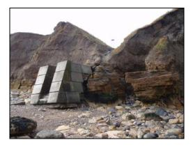
The second failed structure is at the landward end of an outfall to the east of Ryhope Beach Road (pictured, left). Concrete slabs have failed and washed away to expose rubble infill material. The masonry and concrete walls have been outflanked and infill material was being washed out from the structure. Cabinet approval has been obtained to remove the two failed structures in order to close the access at Salterfen and construct a new access at Ryhope Beach Road.
