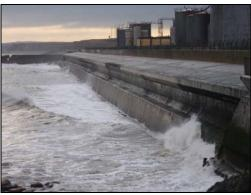
The breakwater marking the southern extent of the Port of Sunderland frontage has failed at the seaward end (pictured, below). A detailed survey of the breakwater is necessary to establish an appropriate course of action. It is likely that the seaward end of the structure is beyond repair so it may be necessary to remove the damaged section and make good the remaining structure.
