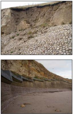
The lower concrete wall fronting Marine Walk is in very good condition (pictured, left). Towards the southern end of the asset there is an older concrete wall supported by the lower wall. This structure was in fair condition with cracks and damage to the crest in places.
