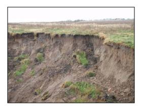
There are two failed structures within the undefended length of frontage. A set of concrete steps providing access to the foreshore from Salterfen Lane, south east of Grangeown has been outflanked and cut off from the cliff behind (pictured, right). The steps have been displaced and now appear to be acting to exacerbate scour to the natural cliffs to either side. Signs at the top of the access inform members of the public that the structure is not to be used.
