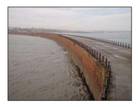
There is a small beach retained between Roker Pier and the Old North Pier. The defences between the two structures consist of a low masonry and concrete seawall and a concrete seawall fronted by a rock armour revetment. The car park to the rear of the concrete seawall contains concrete splash walls. All the assets were in good condition. An additional degree of protection is offered by the high beach levels in this area.
