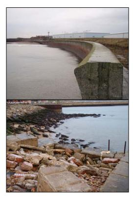
There was an area of sand and shingle foreshore between the seawall and the New South Pier (pictured, below left). The New South Pier (pictured, below right) appeared to be in good condition with minor mortar loss between masonry blocks and minor cracking to concrete elements. The pier provides important shelter to the harbour entrance and therefore should be regularly monitored and maintained.
