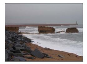
South of the groyne, the rock revetment is interspersed with short lengths of masonry, concrete and sheet piles which appear to have been a part of the North East Pier. The rock volume could be topped up around these structures to improve the standard of defence.
