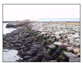
The tie-in between the two defences is in poor condition as there is no crest wall (pictured, right). Here the infill behind the wall is exposed and appears to be becoming washed out from the structure. Loss of fill material may leave the structure more vulnerable as water from overtopping waves will penetrate the rear of the seawall.
