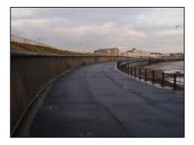
There is some local damage to the grouted stone revetment to the rear of the promenade (pictured, right). Voids are opening up, with water collecting inside the revetment. These voids should be infilled to prevent the voids widening and erosion of the fill material, which could compromise stability of the revetment and the embankment above. The low concrete wall in front of the revetment is cracked with evidence of significant spalling. These sections of wall should be replaced/repaired.
