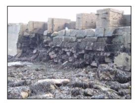
The South West Breakwater requires extensive remedial work and the North East Pier requires major refurbishment or possible replacement, although the importance of maintaining the South Outlet may not be significant enough to justify the capital expenditure. The structures do, however, provide important coastal defence to the area of old dock land forming a barrier between the sea and the Hudson Dock.
