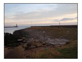
The northern face of the structure is formed by a grouted stone revetment (pictured, left). Several masonry blocks were missing, with concrete patch repairs to the surface which were showing signs of erosion. The southern face of the structure is constructed from masonry, with timber piles also visible (pictured, right). The masonry at the landward end appeared to be in fair condition with the need for some repointing and replacement of missing blocks.
