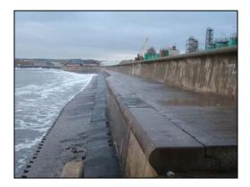
To the south of the outer South West Breakwater the sea defences consist of concrete seawalls with concrete walls set back from the crest which are generally in good condition.
